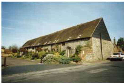
Fig. 18: The former Manor Barn
